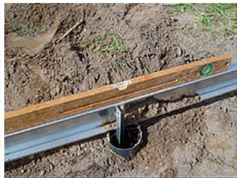
Level the base and check the diagonal measurements again to ensure that the base is level and square.
