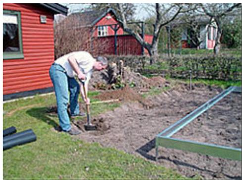
Dig or drill the holes for the ground anchors to be connected to the ground. The holes should be deeper than your frost depth.
