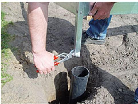
Before you put the ground anchors into the pipes you have to bend the ends outward for best hold in the concrete.
