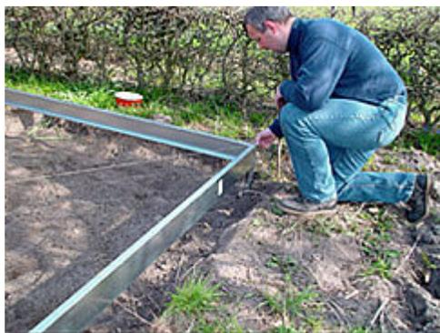
Measure the base diagonal. The measurement must be the same for both diagonal measurements. This ensures that the base is square.
